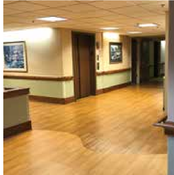
A new flooring detail was added to the Skilled Nursing Facility flooring in key areas.
