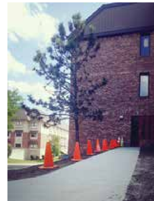
Concrete repair work was completed in early September.
